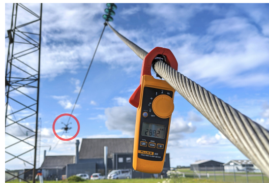
Fig. 11: Powerline 50 Hz 288 A AC current during testing.
